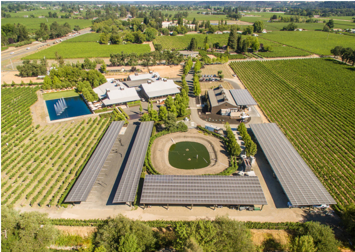
Alpha Omega solar panels shade the crush pad, parking lots and equipment.
